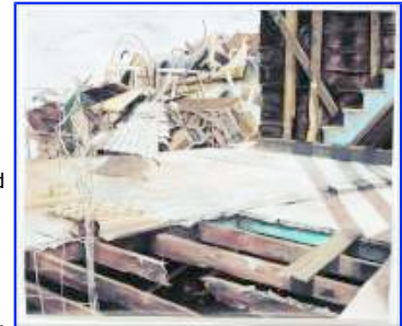
Witness is extrapolated from one of the photographs Ehryn Torrell took of a north-end Halifax house as it was being demolished.
